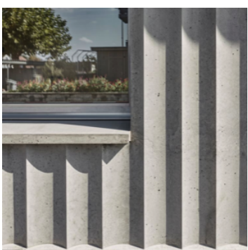
8. PRE CAST SCALLOPPED CONCRETE PANELS WITH 40mm GREY TRAVERTINE CAPPING, SHOP FRONT
