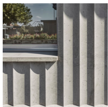
8. PRE CAST SCALLOPPED CONCRETE PANELS WITH 40mm GREY TRAVERTINE CAPPING, SHOP FRONT LOWER WALLS
